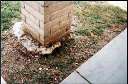
The cracks in the soils are a classical sign of clay soils, which shrink significantly when they dry out. The soils shrinkage cause the piers to settle and lean.
