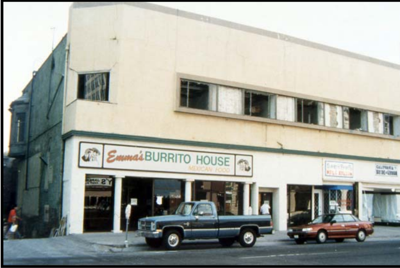
This commercial fire in downtown Sacramento gutted a city block.
