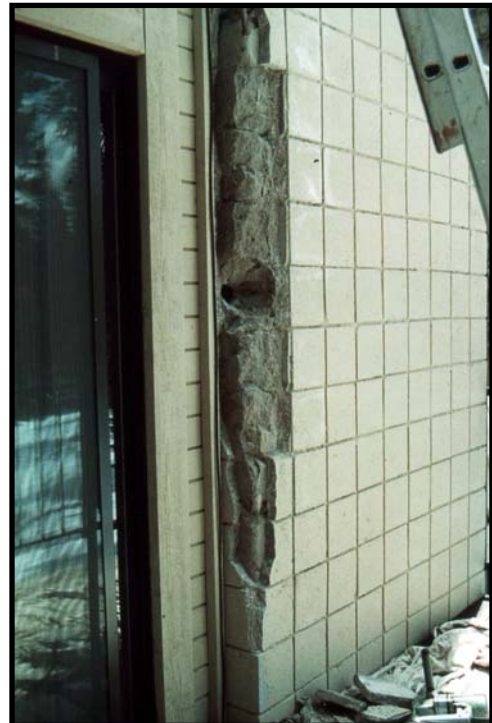
4. This entire piece came off with one blow from a chipping hammer.
